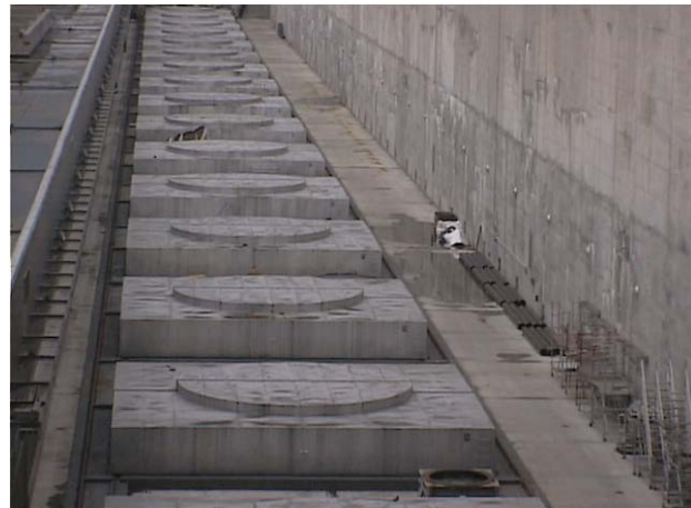
Figure 12 - New generator roof deck roadway, laydown areas and walkway
