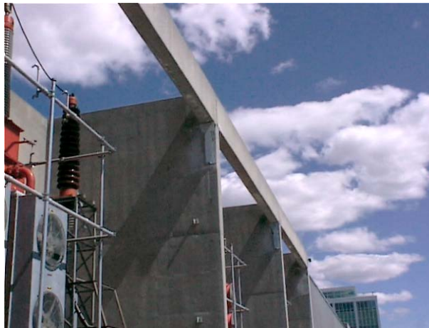
Figure 15 - Transformer bay beams and new steel brackets
