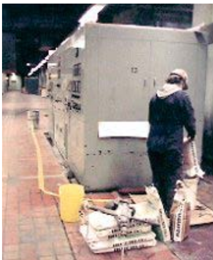
Figure 7 - Preparing to grout around a governor cabinet
