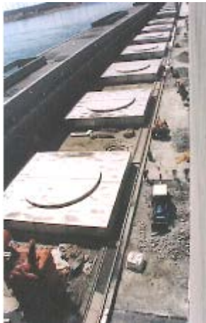
Figure 11 - Generator roof deck roadway and laydown area concrete removal
