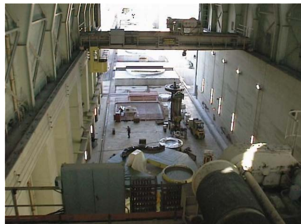
Figure 10 - New erection bay floor
