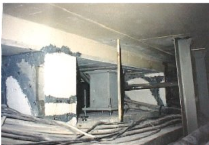
Figure 8 - Structural grouting of columns and new steel column support
