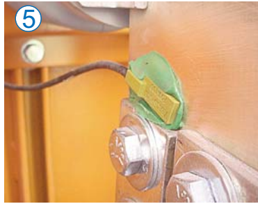
5 FOT - Fiber optic temperature sensor for knife switch temperature monitoring
