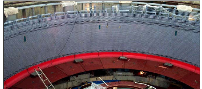
Figure 1: Air gap sensors mounted around the stator wall perimeter.
